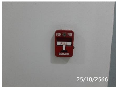
Fire Alarm Manual Station
