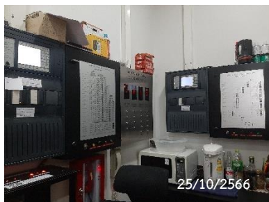
Graphic Annunciator Fire Alarm System
